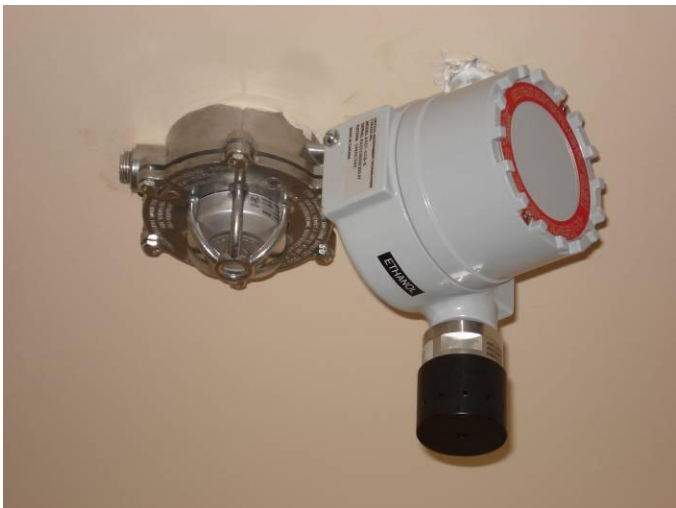
Figure 10. Electrochemical Sensor, with a gas alert alarm. Figure 11. Explosion-Proof Heater.
