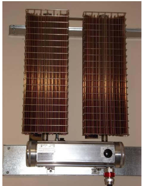
Figure 10. Electrochemical Sensor, with a gas alert alarm. Figure 11. Explosion-Proof Heater.
